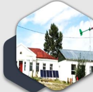
5 kW combined solar and wind power station
